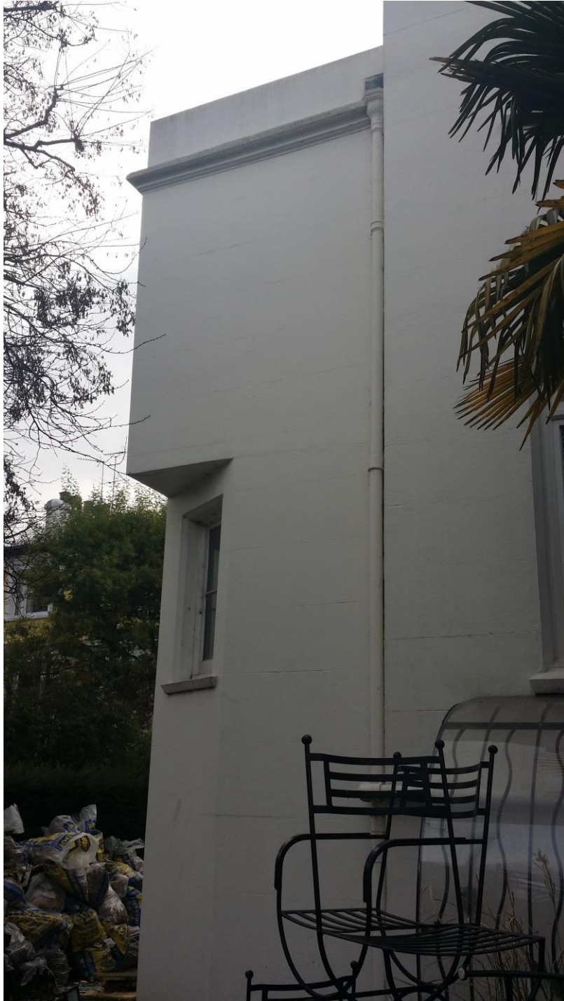
Side of existing three storey rear extension
